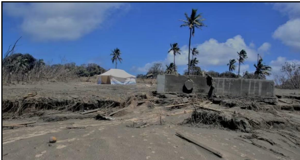
Figure 4: A destroyed home in the island of Mango after the Volcanic Eruption and Tsunami in January 2022.
